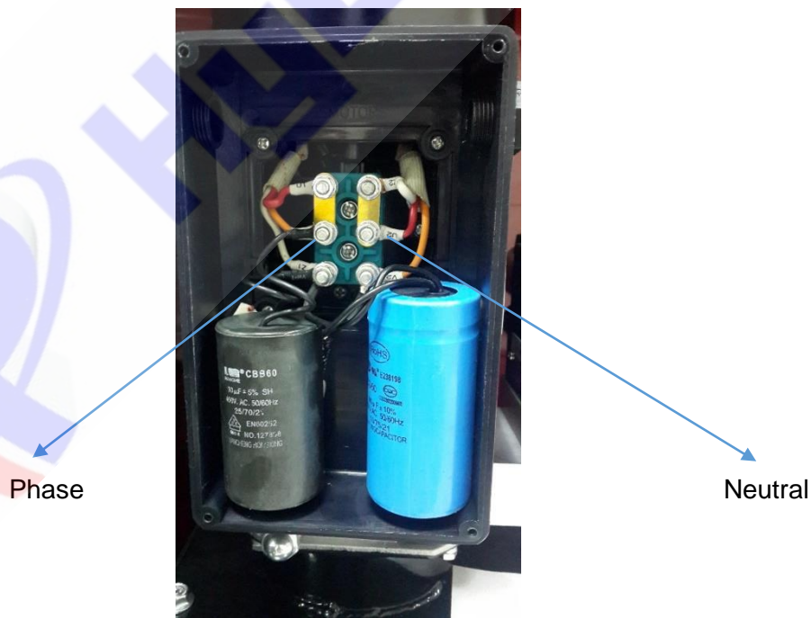
Photo 5. Connection on 220 V AC mono phase motors*
